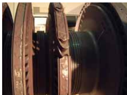
图 10 围带铆钉损伤状态 Fig.10 Damaged rivet
